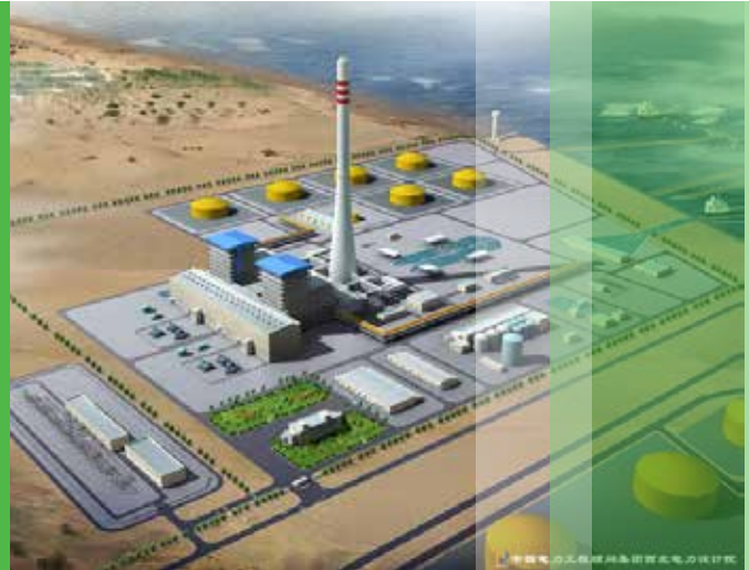
The Rabigh IPP Oil Fired Power Plant, Saudi Arabia.
