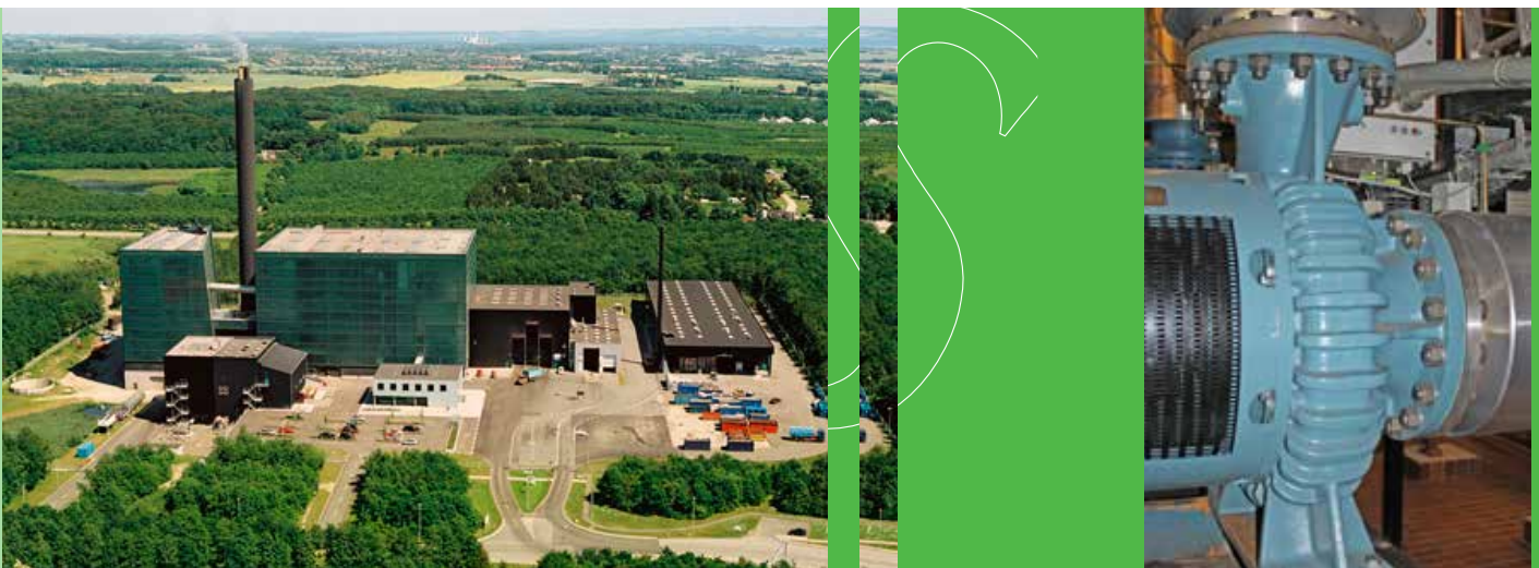
AffaldVarme Aarhus, Waste-to-Energy Plant.
