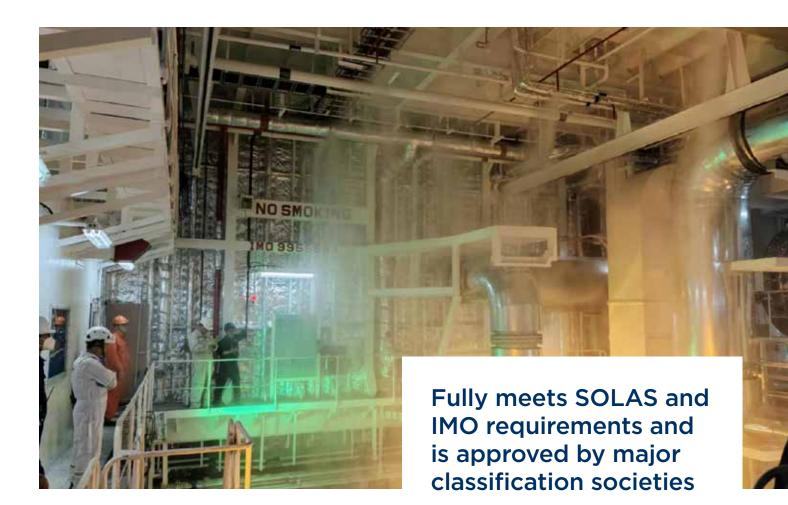
The FineFog<sup>™</sup> local application system lets you protect high-risk objects in accordance with SOLAS requirements without having to shut down the engine and evacuate personnel. Its fire suppression or extinguishing function is based on water mist nozzles complemented by DESMI design for easy and safe operation during the entire lifetime of the product.
